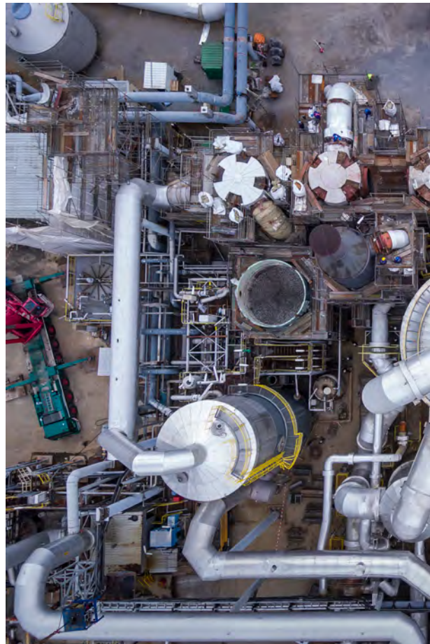
A logistical and technical feat: the successful maintenance shutdown in Pirdop.
